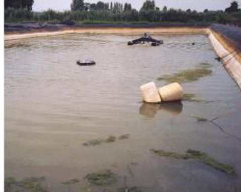
Situation in the basin after 2 weeks; to accelerate the killing of the algae a VitaFloat is added
